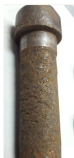
Deep Pitting Corrosion on unloaded side of pin
