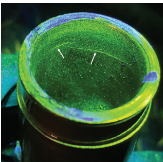
Fluorescent magnetic particle inspection of crack in hollow pin
